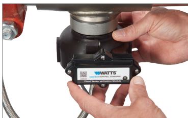
6. Check that the module is fully seated to seal the O-ring and to make electrical contact.
