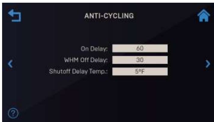
Figure 8-8: Operating Controls: Anti-Cycling Control Screen
