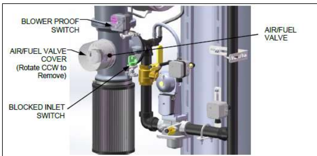
Figure 6-10: Air/Fuel Valve Cover Location
