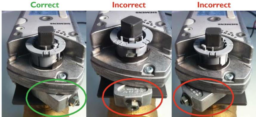
2. To adjust the armature position, depress the actuator manual override button (see below) and turn the armature to the "Correct" position shown above.
